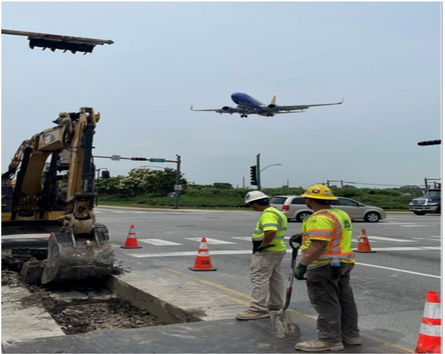
Digging a trench to install 18" main at 55th and Central.
